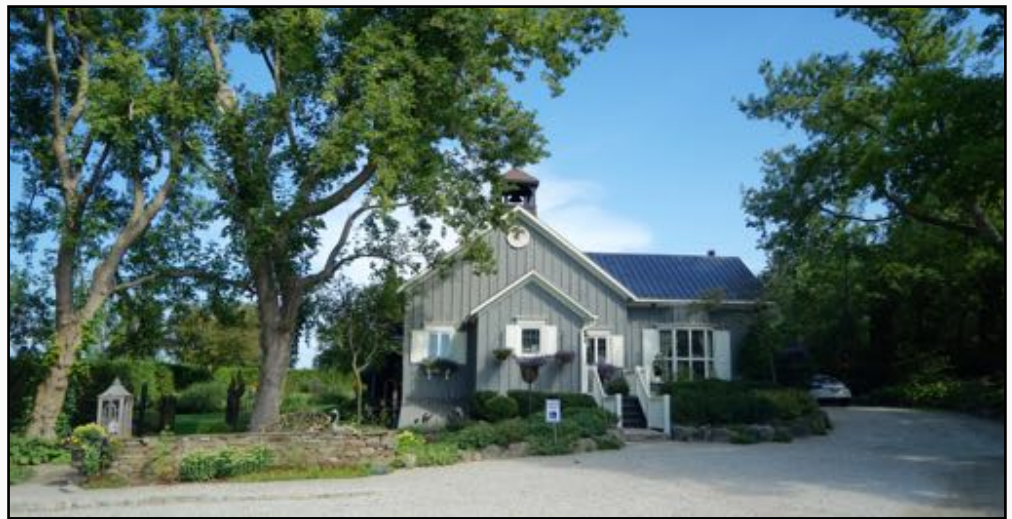
Mrs Mitchell's Restaurant began life in 1889 as Mulmur Township School Section 2 which eventually closed in 1969. In 1980 Maureen Baufeldt opened a restaurant here and named it in honour of the school's last teacher, Mrs Mitchell.
